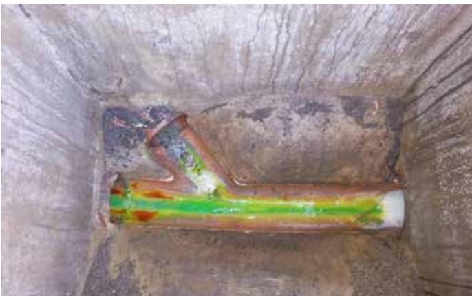
4. Carefully dig a trial hole or trench to locate the pipe.
