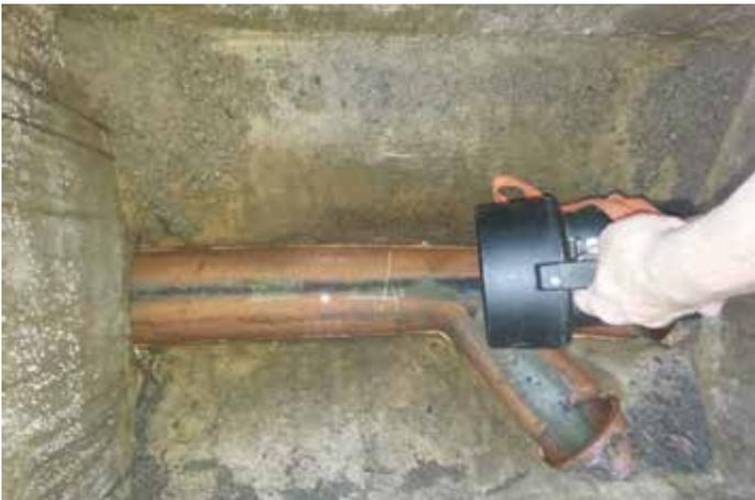
3. Rod the sewer or drain from the manhole or inspection chamber.
